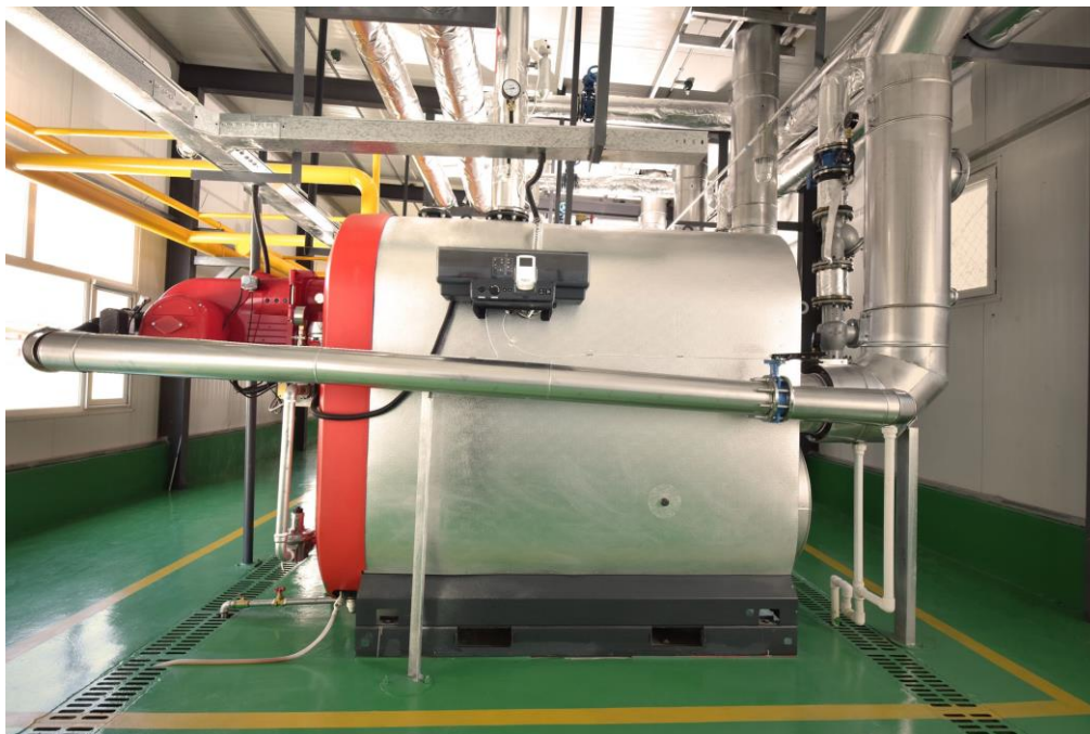
Extremely low nitric oxide emissions: The optimised Bosch heating boiler system with recirculation technology.
