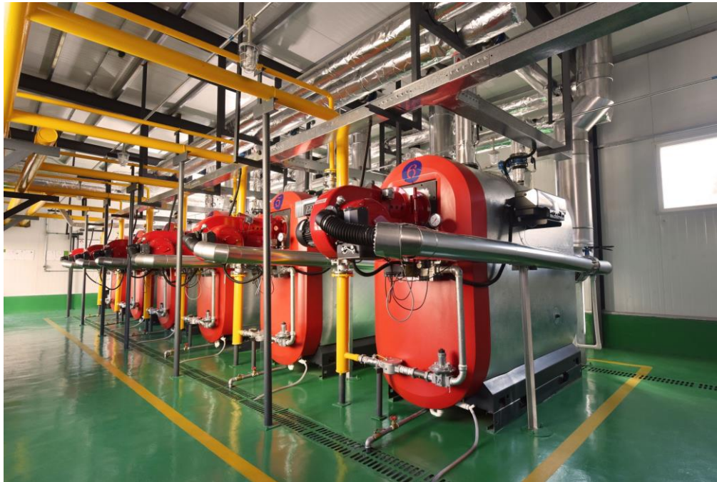
Part of the Uni Condens heating boiler systems from the first order in 2016 – each boiler generates 1.2 MW heat.
